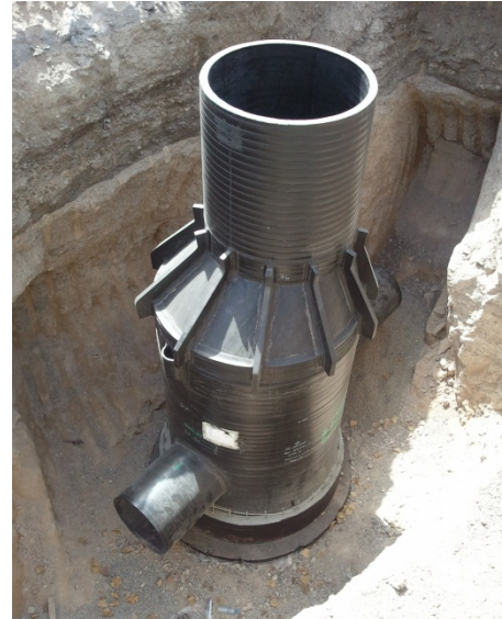
Pic 1: PE100-Manhole for Sewer DN1600/1200 (Source: UGPM, Sultanate of Oman)
