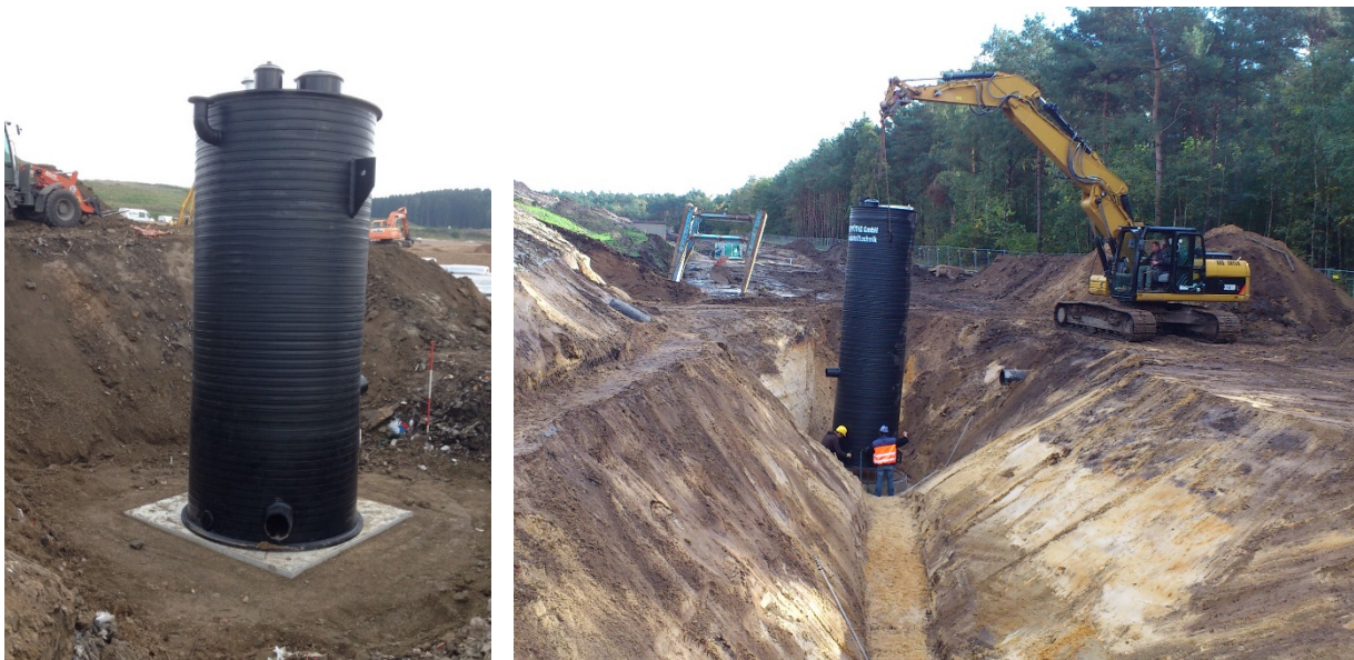
Pic.3: Manholes in Landfill application (Henze GmbH, RBV Pöthe, Germany)
