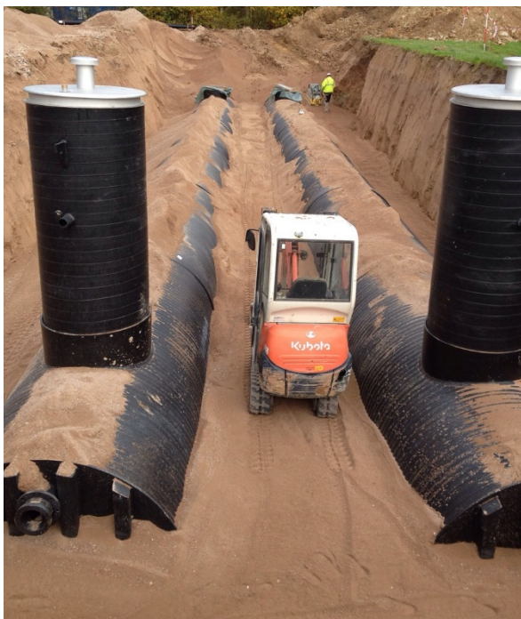
Pic. 7: Double wall Leachate-reservoir (Henze GmbH, RBV Pöthe, Germany)
