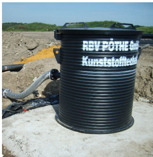
Pic.6 - Gas-well-manhole (Henze GmbH, RBV Pöthe, Germany)
