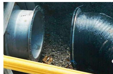
Connection PEHD/Stainless Steel
