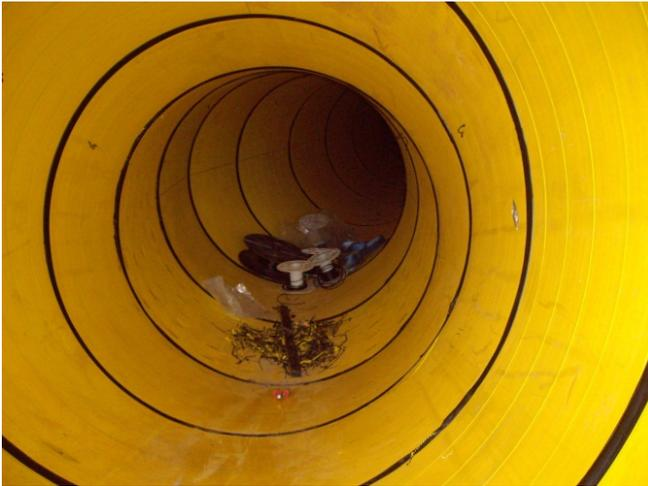
Image 9 - Installing of 1250mm segments into the closed pipeline under the transformers
