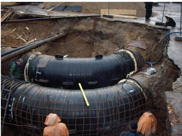
Image 8 - Preparing of the 60 degree bends for concrete supports
