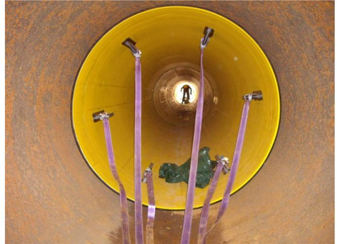
Image 7 - Stubs for anchoring the pulling ropes and spreading
