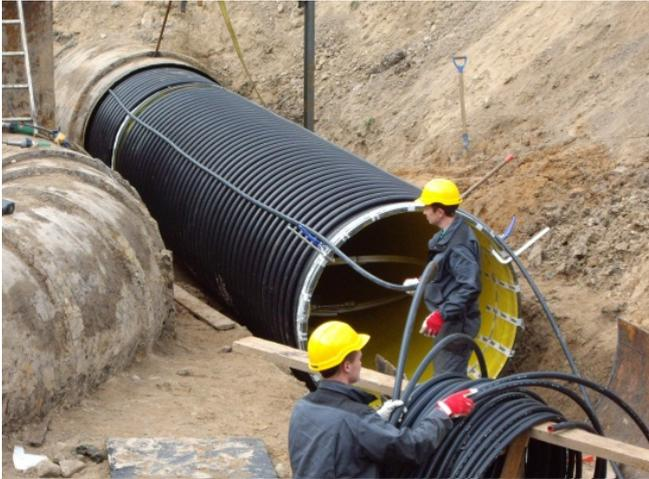
Image 6 - Start point of the relining, Kraih electro-fusion welding and bentonite pipe installation
